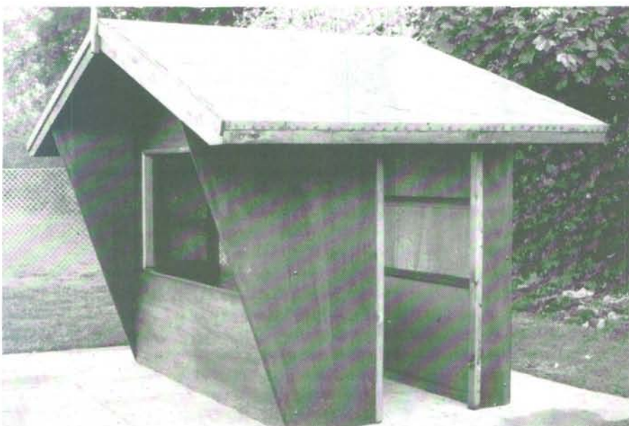
The design and construction of a play shop for a primary school in Sidcup. Work was done on this project by Ossie O'Garro, Alan Brown, Trevor Southee, Alan Thredder, and Martin Pentecost.
